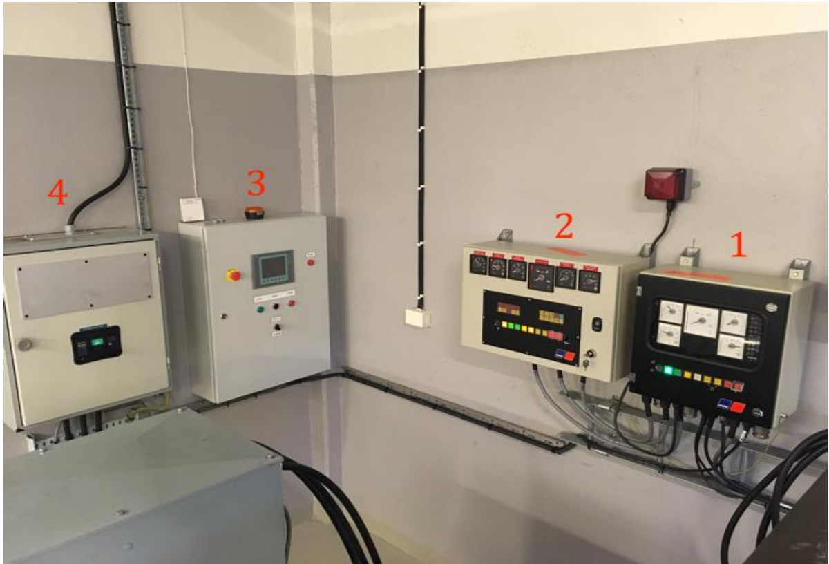
Figur 7. 1. Local Operating Panel (LOP) 2. Main Control Stand (MCS) 3. Remote Control Stand (RCS) 4. Lastbryter
