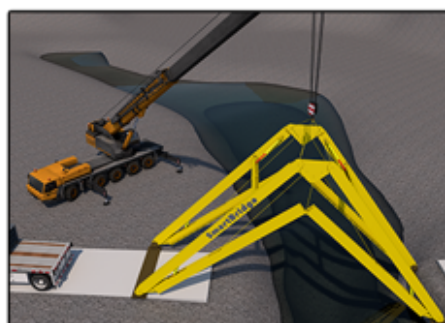
The Tec-Trans container based Smartbridge is 20-32 meters long, 4 meters wide and built for loads over 100 tons. Photo: Tec-Trans
