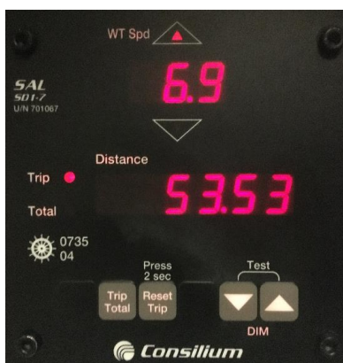
Figure 12: HMI Electromagnetic Log
