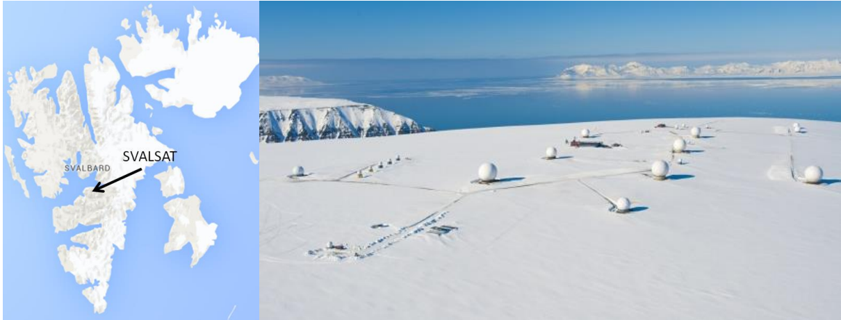
Figure 3.4 KSAT Svalbard Satellite Station at Svalbard (Extracted from: www.ksat.no )
